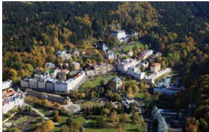
View north to the spacious 'spa in a park'
