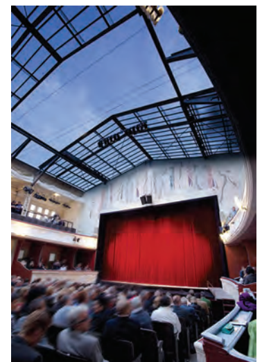
Retractable glass roof of the historic Sommerarena enables seasonal performances under open skies
