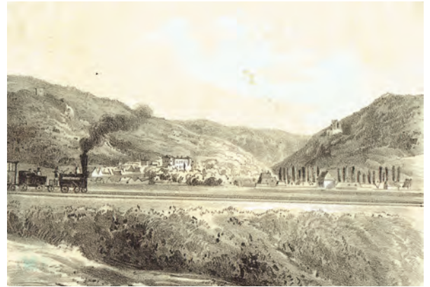
The Sudbahn Railway, Baden bei Wien . In the background are the two ruins Rauhenstein and Rauhenneck framing the entrance into the therapeutic landscape “Helenental”
